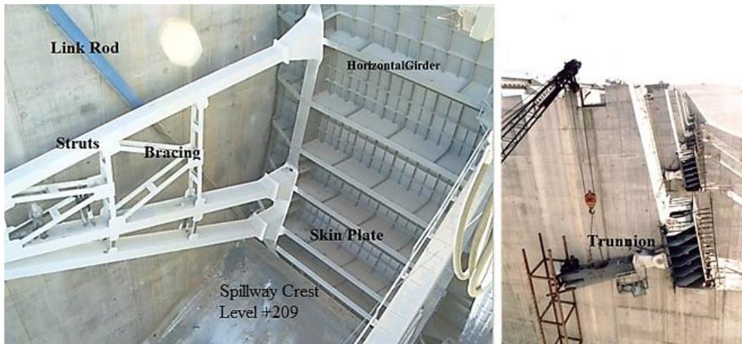
Fig. 3 Primary radial gate components, Karkheh Dam
