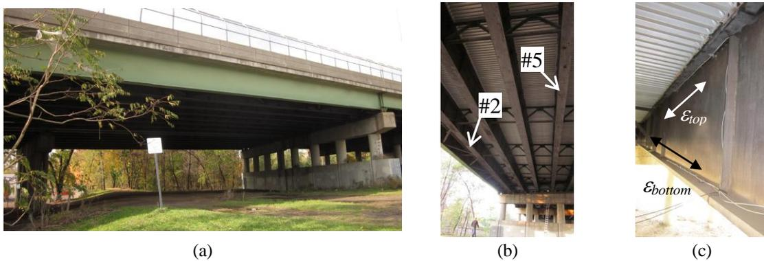
Fig. 1 US202/NJ23 overpass consisting of concrete slab supported on steel girders. General side view (a), detail of steel girders #2 and #5 under the concrete slab (b), detail of the sensor positioning at the top and the bottom flange where longitudinal strains are collected, respectively  $\epsilon_{top}$  and  $\epsilon_{bottom}$  (c) (Sigurdardottir and Glišić 2013)
