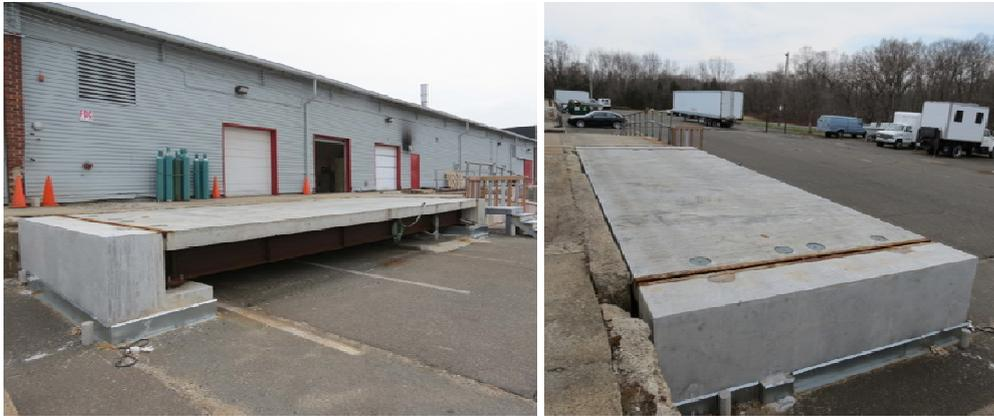
Fig. 7 NDE validation bridge structure
