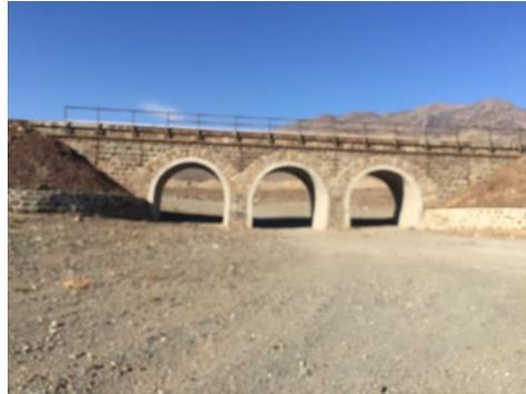
Fig. 6 A typical retrofitted masonry arch bridge by sprayed concrete technique in Iranian railway network
