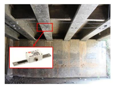
Bridge information: Name: Pawiro Baru A Bridge type: PCI Girder Spacing of girders: 1.55 m Length of span: 12.00 m Number of girder: 6 Overhang width: 975 mm Construction: 1994
