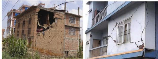
Fig. 2 Failure of masonry wall during an earthquake (source: Tripathy and Singhal 2021, Asian News International)
