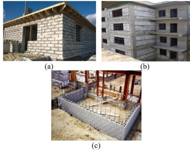
Fig. 1 Types of Masonry walls: (a) Unreinforced masonry walls, (b) Unreinforced masonry infill walls and (c) Grout-reinforced masonry walls
