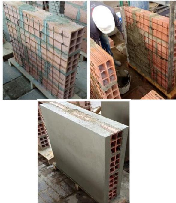
Fig. 4 Strengthening of URM walls using wire mesh and plastering using mortar. (Source: Sandoval *et al.* 2021)
