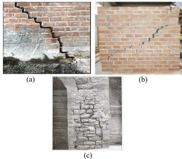
Fig. 3 The local failure mode of URM: (a) detachment failure, (b) detachment fractures alternate line of sliding, and (c) compression failure (source: Angelillo *et al.* 2014)
