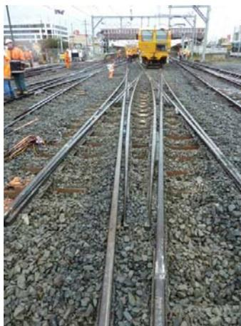
Fig. 9 Double slips installation and resurfacing
