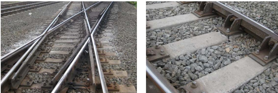
(a) pulverised ballast and broken concrete sleeper due to poor energy dissipation of material
