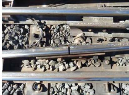
(f) a joint gap at a mechanical joint
