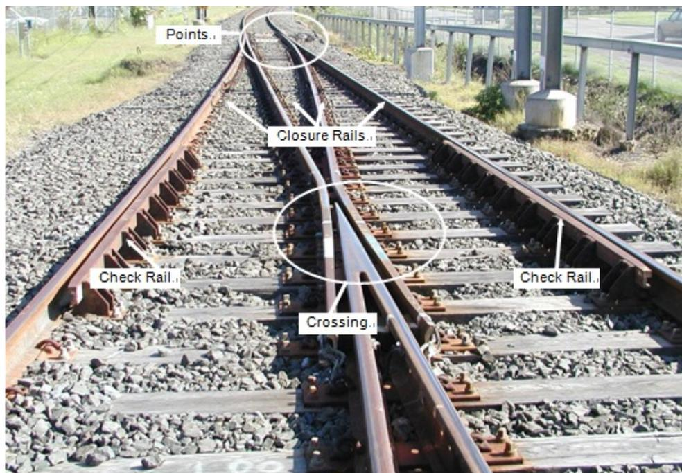
Fig. 1 Typical turnout structure and geometry
