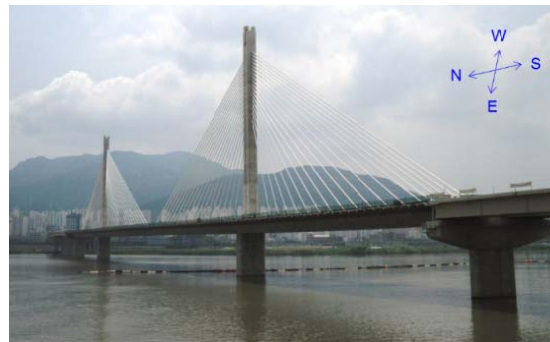
(b) On-site View
