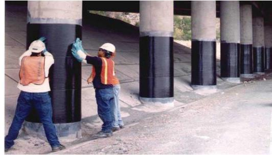
Fig. 2 Strengthening of the bridge piers with FRP layers
