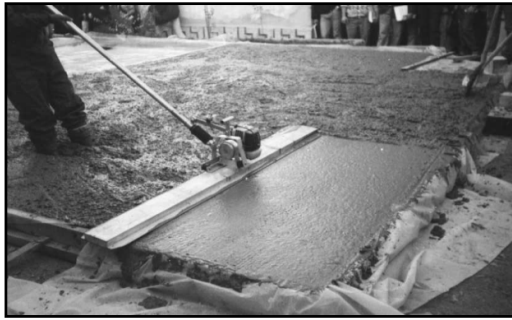
Fig. 1 Compaction of concrete with vibrating screed
