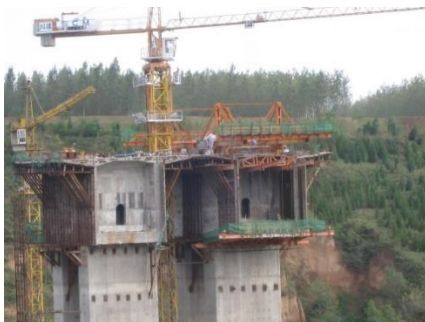
Fig. 3 View of box girder on the pier top
